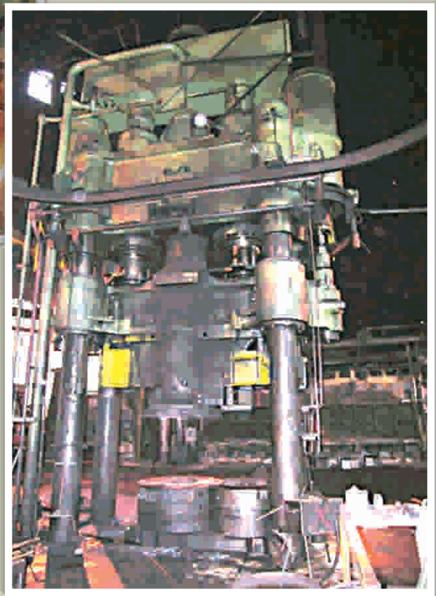
Davy Forging Press under commissioning ▶
